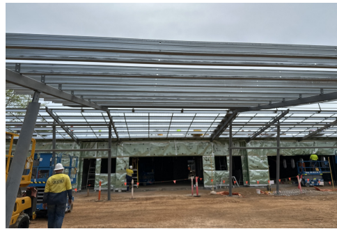
Structural steelwork under installation, new preschool, Parap Primary School NT.
