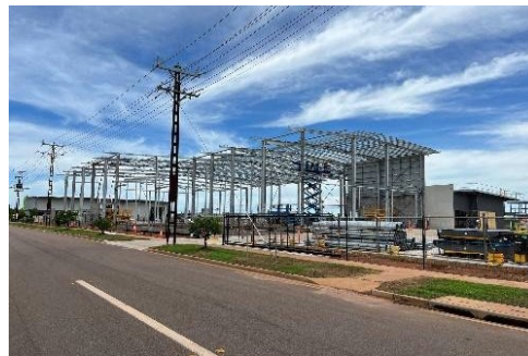
Erected structural steel frame, Tyremax warehouse, Berrimah NT.
