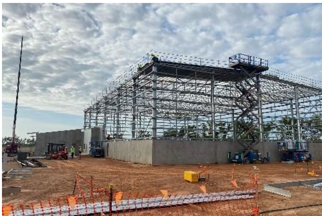
Structural steel installation, APA Group facility, Winnellie NT.
